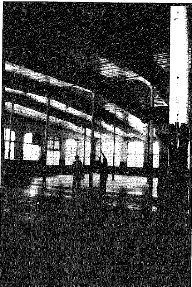
Interior of 210 Pine Street Yarn Mill
