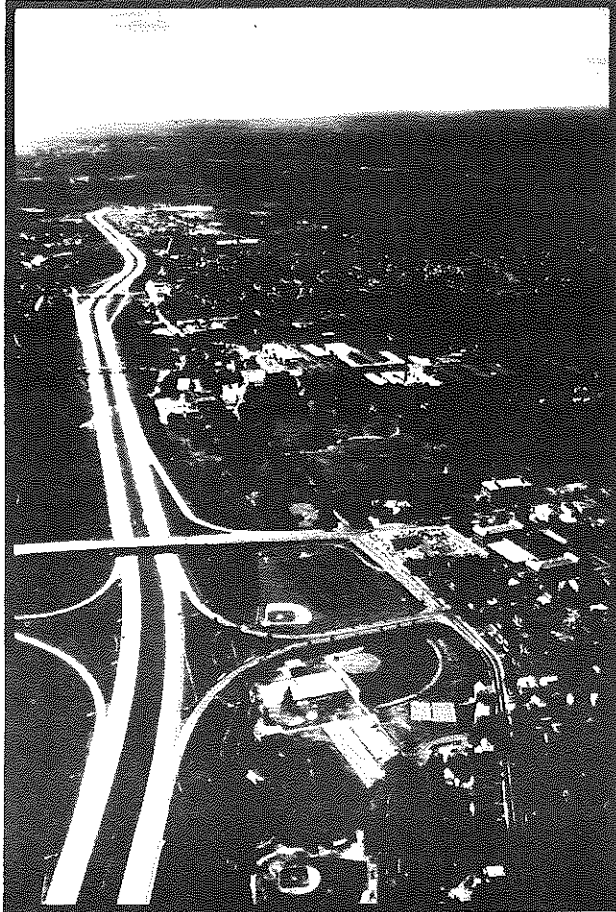
Interstate 84 - View west toward Hartford
